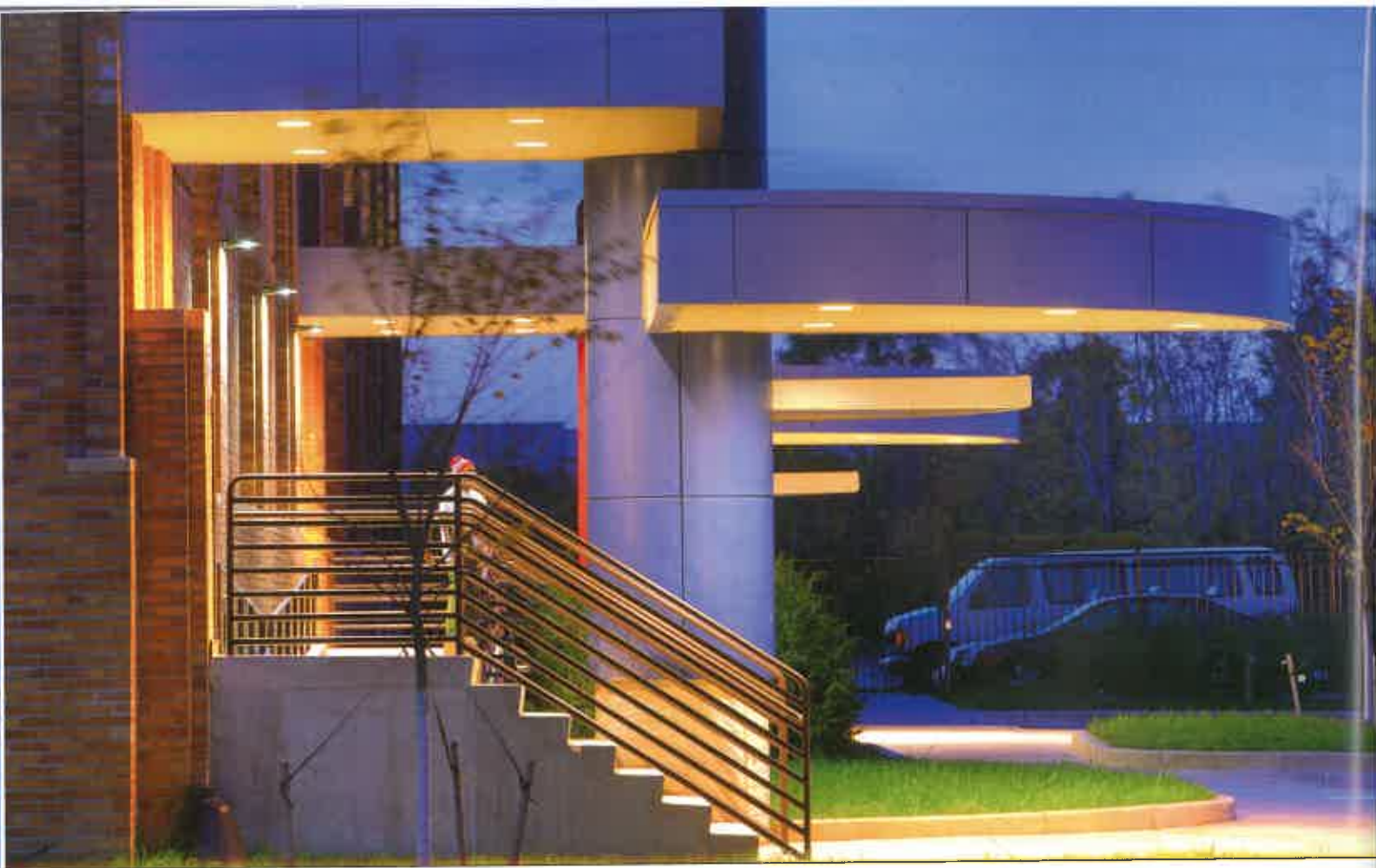
Marked by a contemporary canopy, the new main entry was moved to the east side of the building, both for ADA compliance and to create a single, secure point of access for residents.
